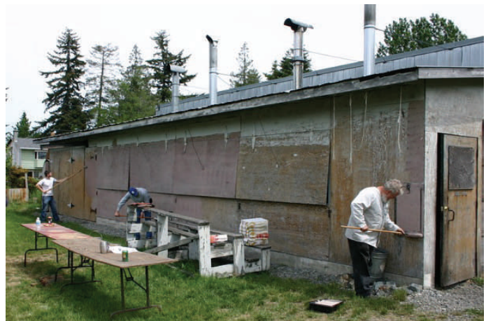
Charlie Low powerwashed and prepped the clubhouse so we could apply the primer coat of paint. It was a mix of several colors that turned out a purplish mud color. The finish coat will be applied as weather permits over the next week. Please thank Charlie for his contribution of time and effort.
