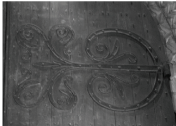
The topmost hinge of 3 on each door at Durham Cathedral; and there's another set of these doors at the other end.
